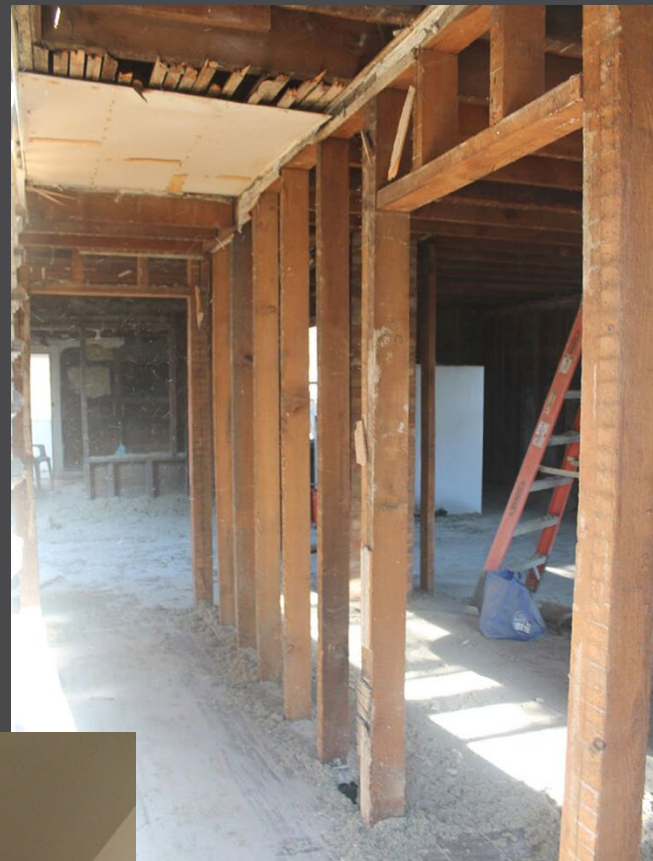
MAIN FLOOR DEMOLITION
