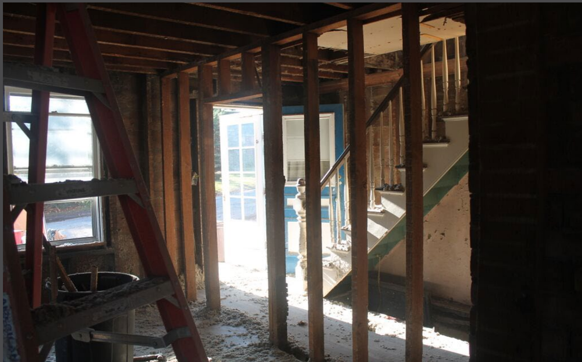
LIVING ROOM DEMOLITION
