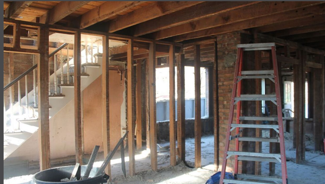
FIRST FLOOR DEMOLITION
